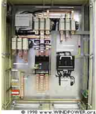
A high voltage section of a controller of a megawatt machine
