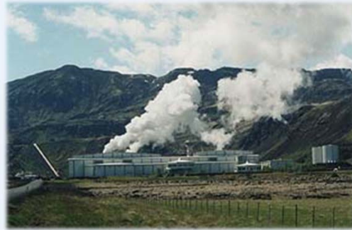
Nesjavellir Power Plant, Iceland; 90 MW
