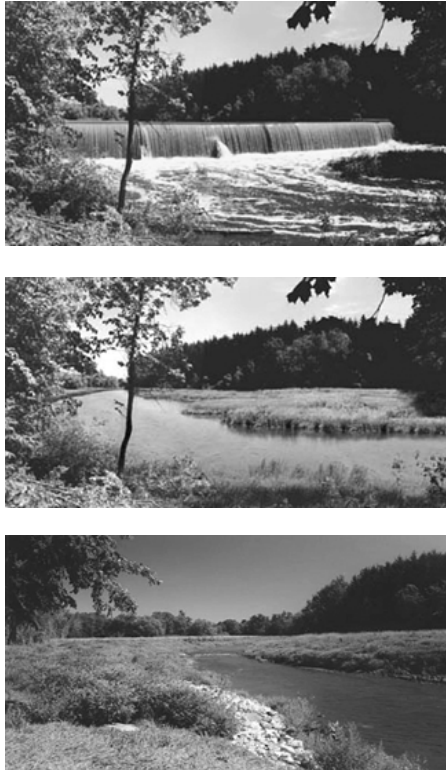
Figure 3.4 Computer simulations help the community visualize a former impoundment after removal. (Top) Photo of Franklin Dam, Sheboygan River, Wisconsin. Source: River Alliance of Wisconsin. (Middle) Computer simulation by a WDNR biologist of the site after dam removal. Source: Wisconsin Department of Natural Resources. (Bottom) Photo of the actual site after 12 months. Source: River Alliance of Wisconsin.
