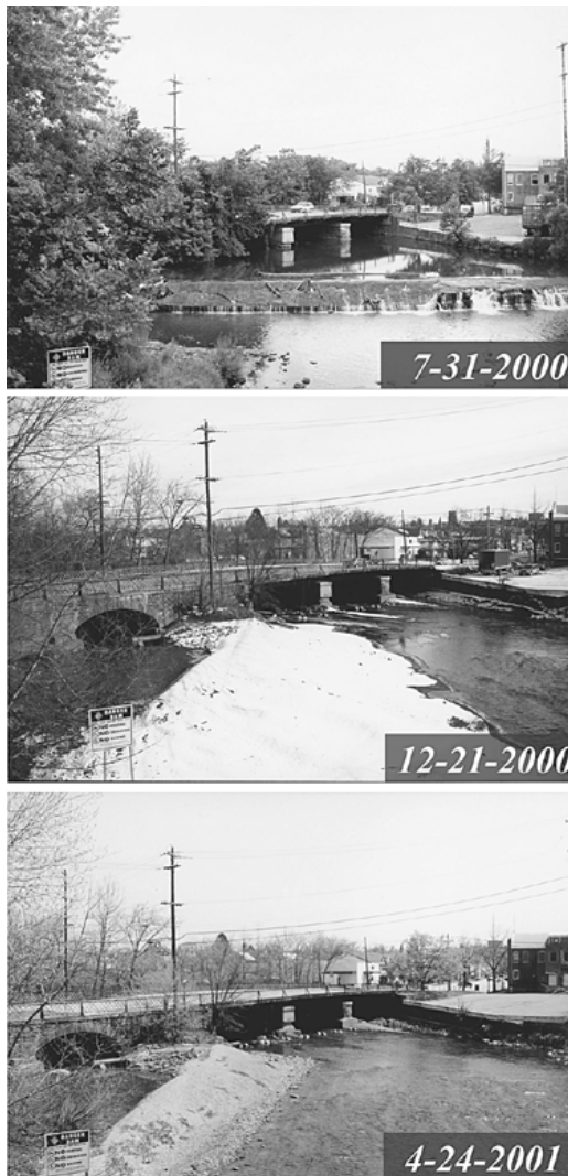
Figure 5.1 Channel of Manatawny Creek before (July 2000) and after (December 2000, April 2001) dam removal. The views are looking upstream directly at the dam. The run-of-the-river dam was about 2 meters in height. After the two-phase removal in August and November 2000, efforts were made to stabilize the left bank of the stream. In mid-December 2000, a significant flow event (2.5-year recurrence interval) caused large amounts of coarse gravel to accumulate at the dam site. With each subsequent runoff event, the bar has been decreasing in size because of sediment migration farther downstream. At present, the right bank area, which has been blocked off from the main channel because of the sediment bar, is a wetlands area. Courtesy of Karen Bushaw-Newton.
