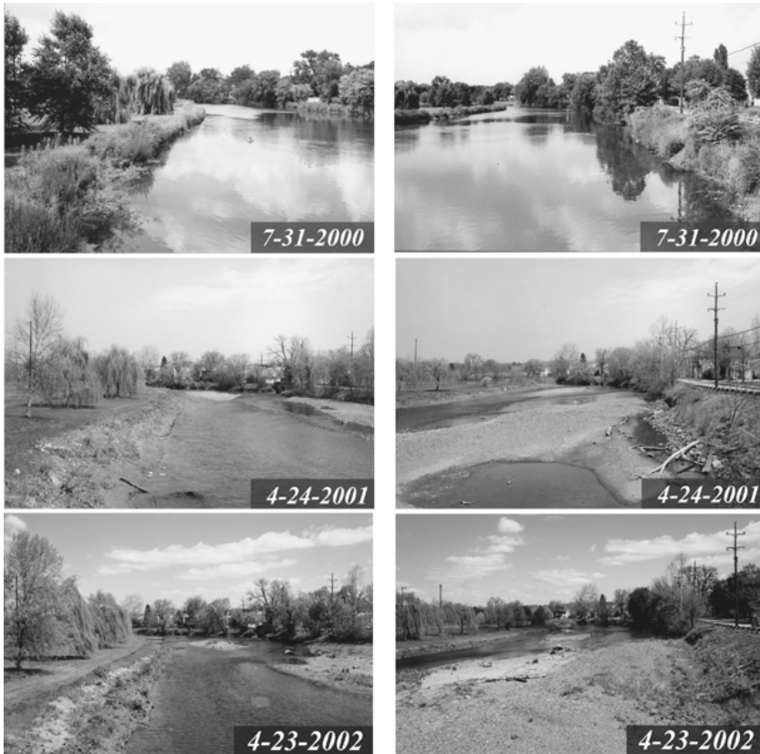
Figure 5.2 Changes in the impoundment area of Manatawny Creek before (July 2000) and after (April 2001, 2002) dam removal (the right bank of the creek is shown in the left-hand column and the left bank in the right-hand column). Prior to removal, water levels in the impoundment were between 1 and 2 meters. After removal, the water levels decreased to less than 0.3 meters in many areas, resulting in exposed banks and a large sediment bar on the left bank. With each major rainfall, coarse gravel sediment has migrated downstream through the former impoundment. Observable in the postremoval photos, a new channel has formed along the right bank of the former impoundment, while sediment has accreted on the left side of the former impoundment. In the fall of 2001, the right bank underwent restoration through regrading and replanting of native vegetation, and the growth is evident in the April 2002 photo. Courtesy of Karen Bushaw-Newton.
